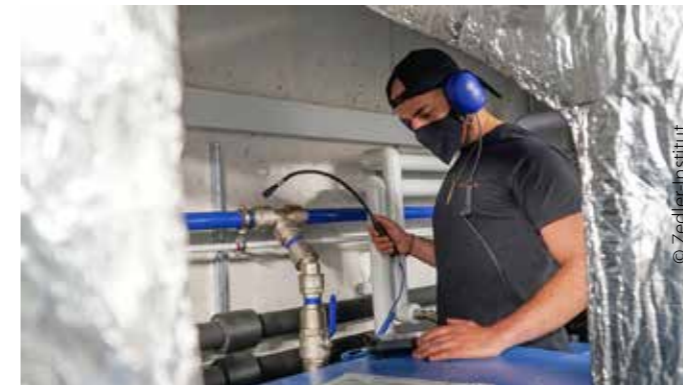
Kevin Togonal checking the compressed air network for possible leakages
