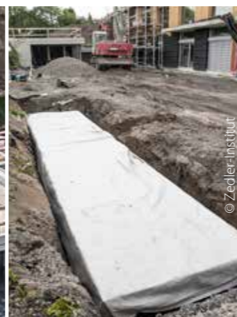
Infiltration ditches for a slow seepage of the rain water
