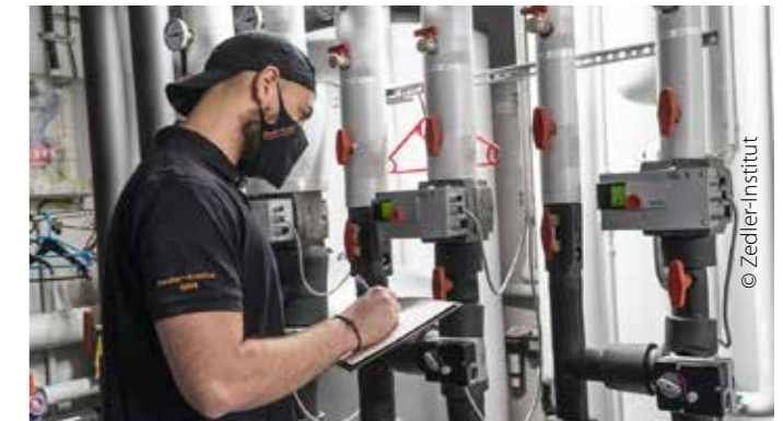
Monthly reading of all flow volume meters, heat measuring devices and power meters
