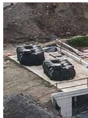
Rain water cistern (two times 5,000 l) prior to installation
